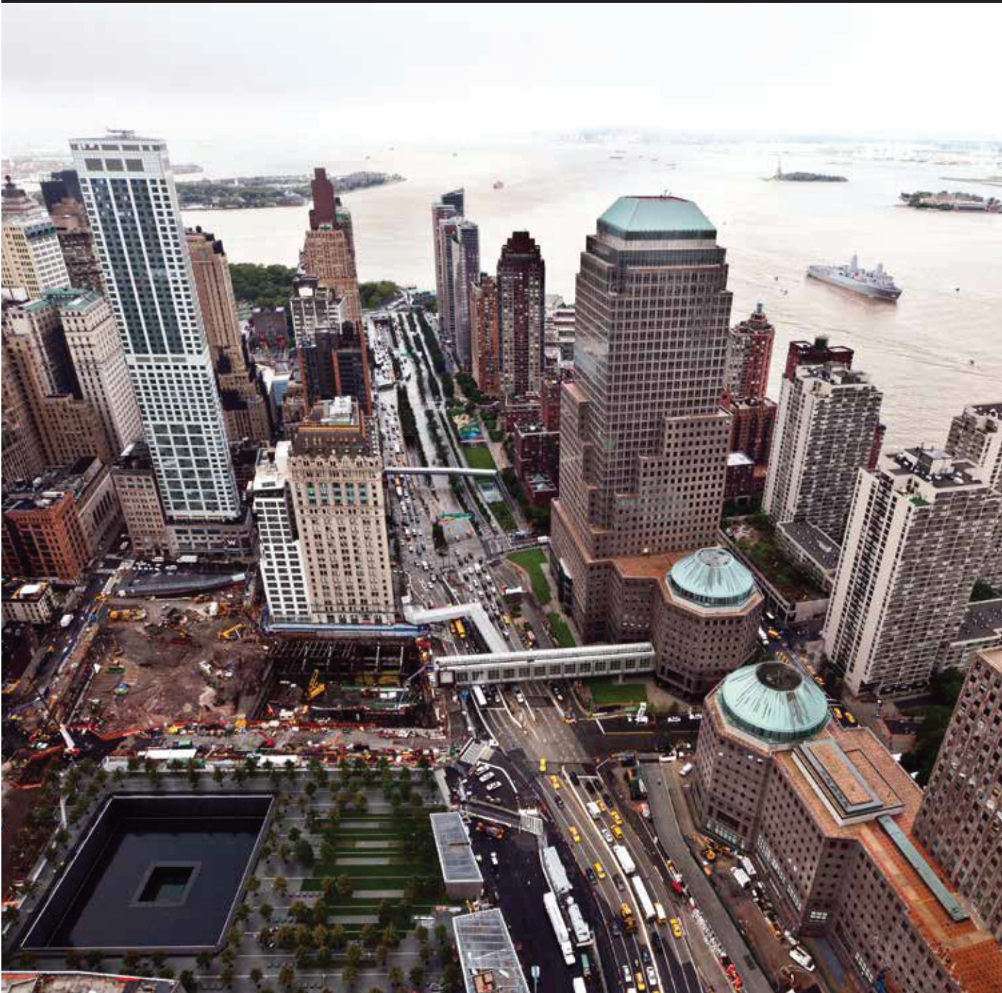
In September 2011, the crew of the USS New York , upper right, man the rails and present honors while passing the National 9/11 Memorial. On board are family members of victims and first responders from 9/11 and Marines from Camp Lejeune. The ship was built with steel recovered from Ground Zero. (U.S. Marine Corps/Randall A. Clinton)
